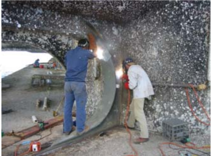
Welding-out 180kg gusset on rig column SC3.
