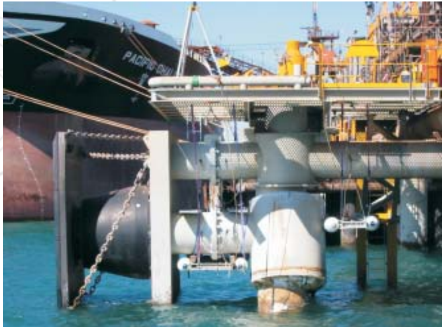
Wharf berthing dolphin with access platforms, rigged in position.
