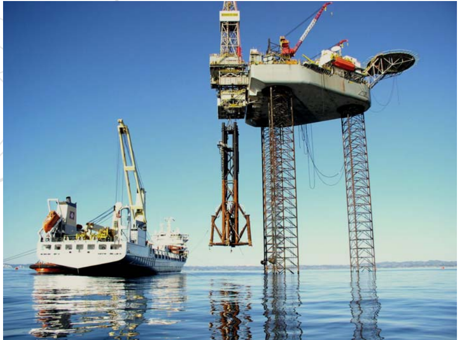
Successful lift of the jacket by the Ensco 56, from the HLV Annegret
