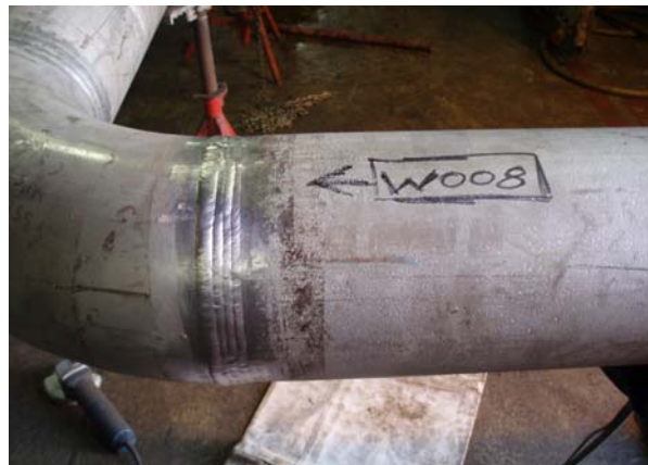
Field weld on 6" sch160 SS pipe awaiting NDT and trachibility recording
