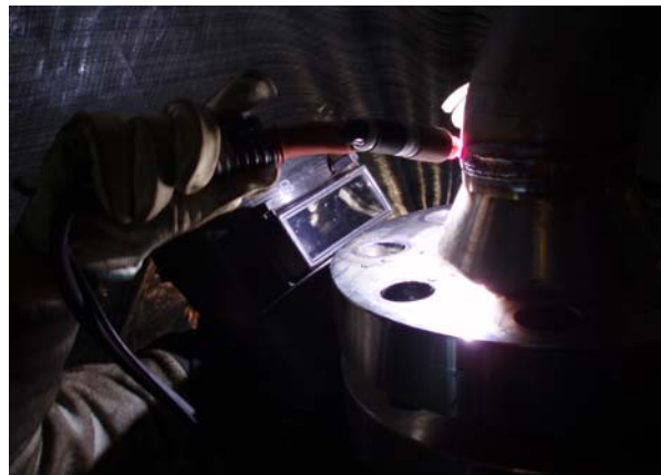
Field weld on derrick being carried out within a welding habitat
